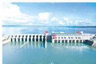
Lower Sesan II Hydropower Station
