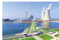
Sahiwal Coal-fired Power Plant
