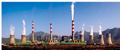
Qinbei Power Plant
