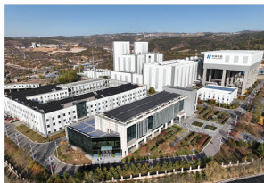
Rooftop PV Power Generation Project of Dongshan Gas Power Station
